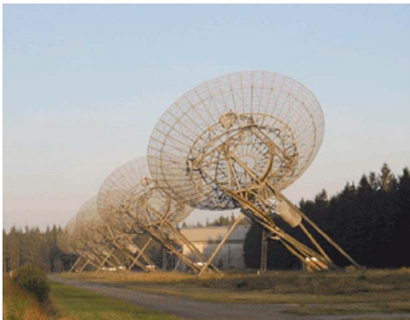
Fig. 7.3. The westerly 5 elements of the WSRT. The fixed antennas are 144 m apart for a total baseline of 1.6 km. The assembly hall is visible in the background. (ASTRON)
