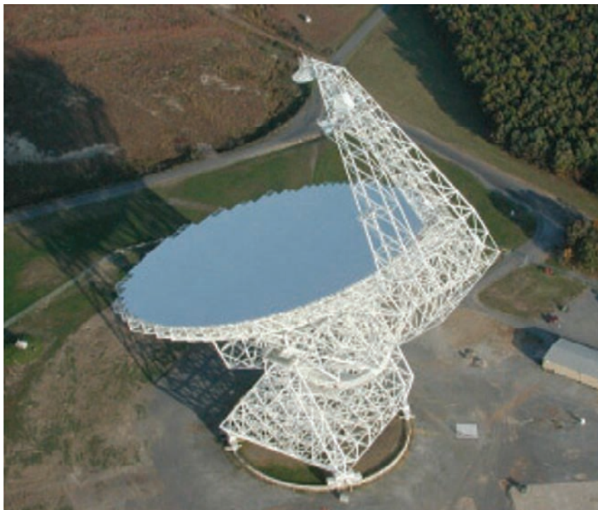
Fig.1.6. The Green Bank Telescope (GBT) of NRAO. This "clear aperture" antenna is an off-set piece of a paraboloid of 100 m diameter and provides a very clean beam with low far-sidelobes. Like the Effelsberg antenna it uses a Gregorian focus arrangement with elliptical secondary reflector. Prime focus operation is used for long wavelengths. (NRAO/AUI/NSF)
