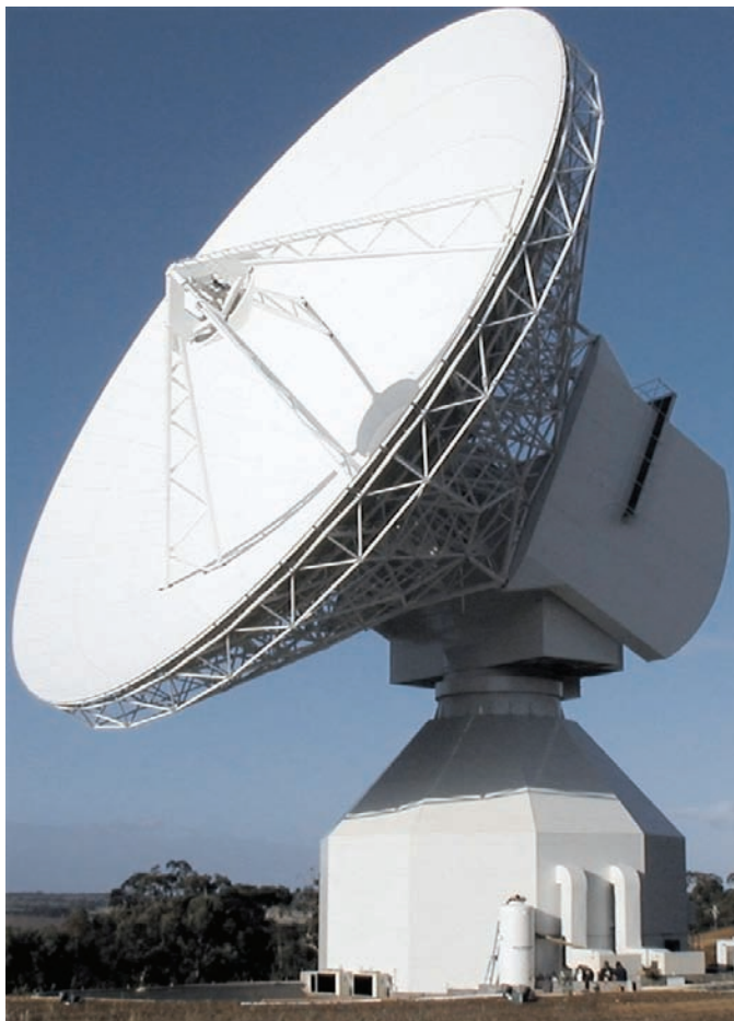
Fig.1.4. Example of a modern deep-space ground station. This 35 m diameter ESA antenna is located in Western Australia and was designed and built by Vertex Antennentechnik of Germany. (ESA/ESOC)
