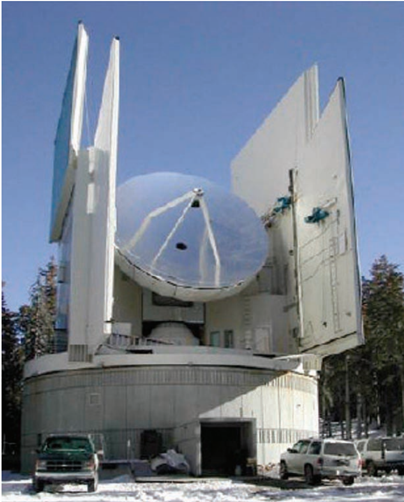
Fig. 7.14. The HHT on Mt. Graham, Arizona. The enclosure rotates with the telescope. Receiver and control rooms are just visible behind the reflector. The doors and roof panels are closed during inclement weather. (Photo by the author)
