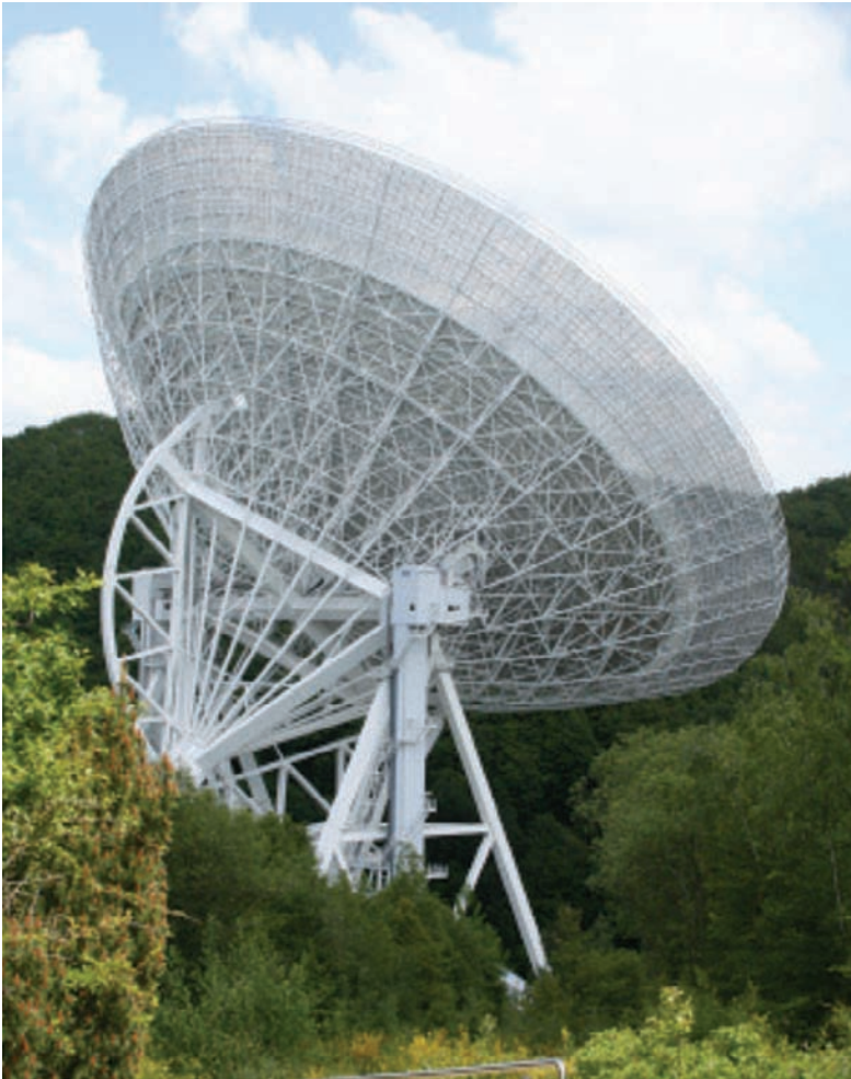
Fig. 7.9. The 100-m diameter Effelsberg telescope of the MPIfR, Bonn, Germany. The "umbrella" reflector support and the rear half of the octahedron structure are well visible. The cabins at the elevation bearings are 50 m above the ground. The collar around the edge of the reflector serves to reduce pick-up of ground radiation. (N. Junkes, MPIfR)
