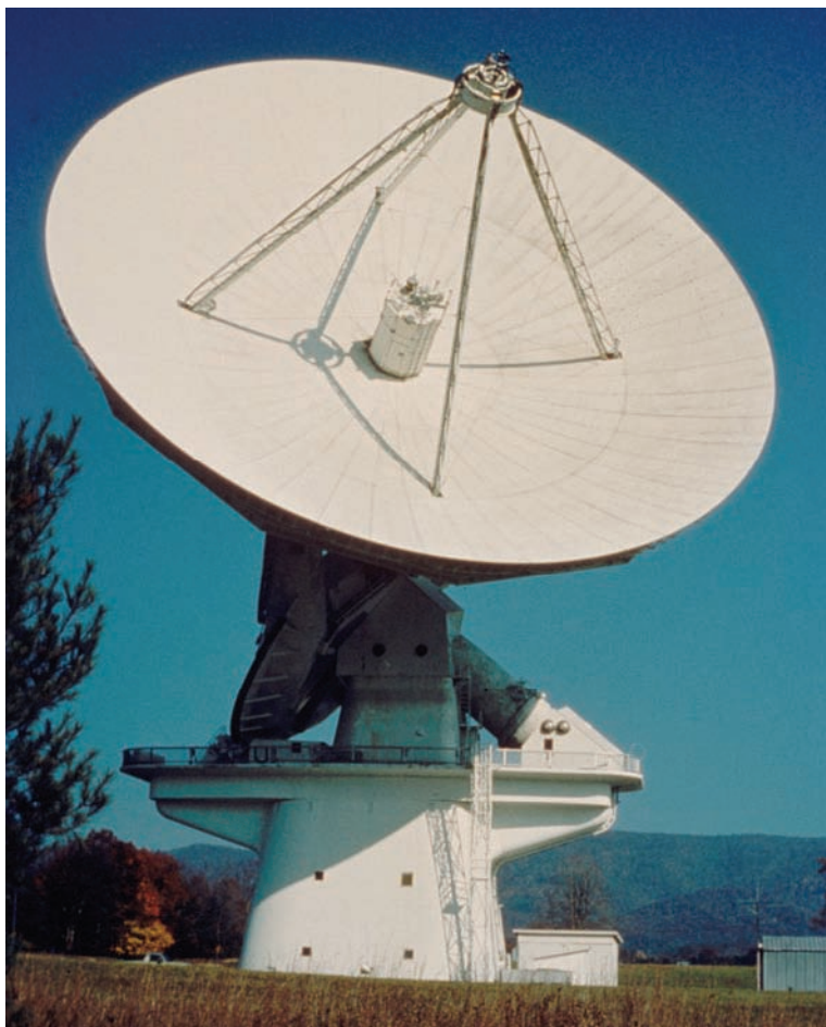
Fig.1.5. The NRAO 140-ft telescope. The polar axis runs on hydrostatic bearings. The reflector structure and panels are made from aluminium. The original prime focus geometry was converted to Cassegrain and the receiver box in the secondary focus protrudes from the vertex of the main reflector. (NRAO/AUI/NSF)
