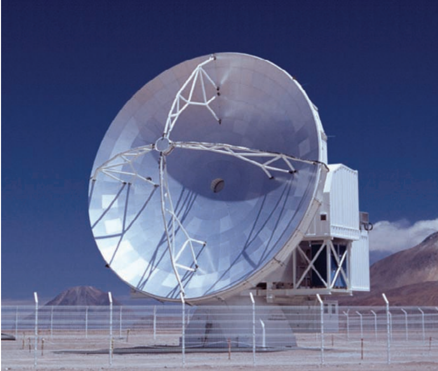
Fig.1.9. The 12 m diameter APEX antenna on the ALMA site in Chile, derived from one of the ALMA prototype designs. To accommodate large multi-feed receivers, the antenna uses a Nasmyth focus with two large equipment rooms at either side of the elevation bearings. (ESO / Max-Planck-Institut für Radioastronomie)
