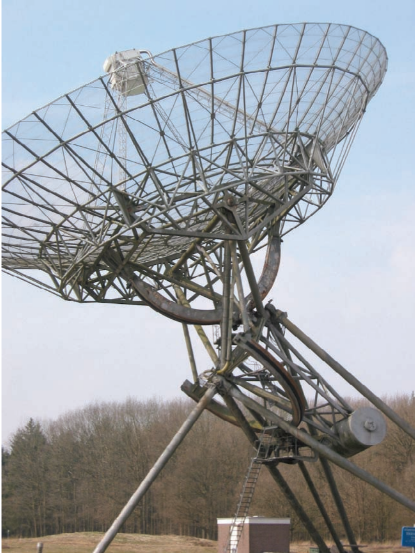
Fig. 7.4. Element antenna of the WSRT with an equatorial mount, a 25 m diameter wire-mesh reflector and primary focus receiver box. After setting up the base pentapod, the assembly required only 4 lifting maneuvers to complete the antenna, (Author's photo)
