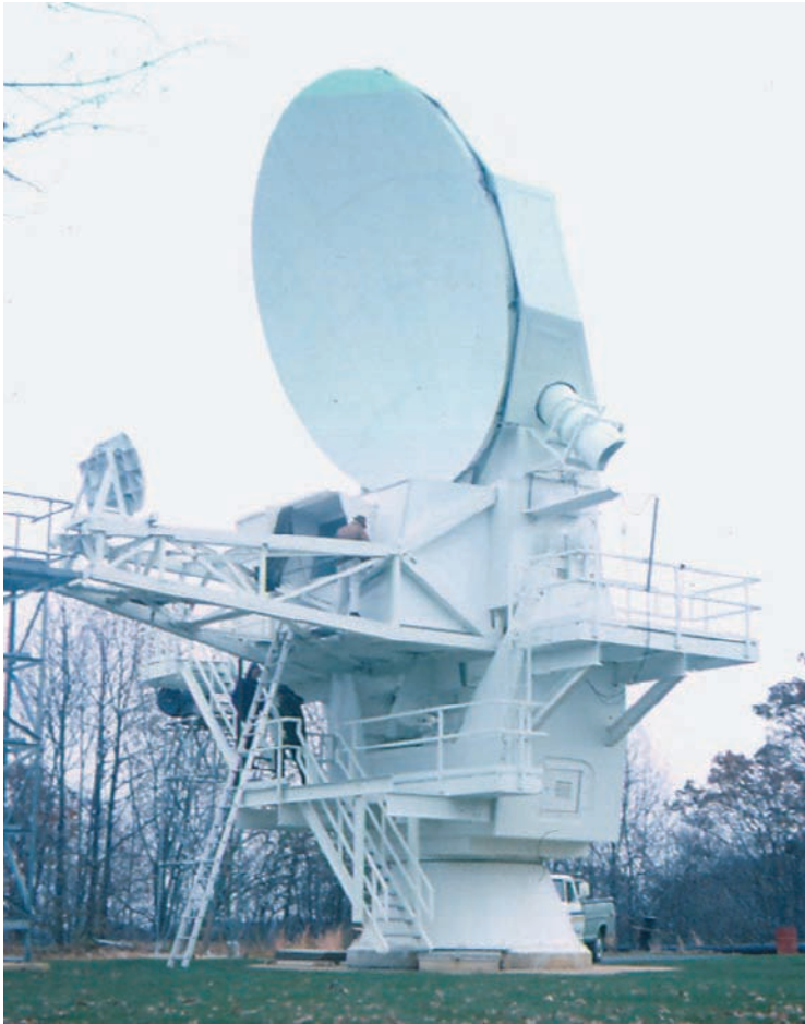
Fig. 6.17. The Bell-Laboratories 7-m Offset-antenna at Holmdel, NJ, USA. Subreflector is to the left; The person is entering the feed- and receiver-cabin under the main dish. (Photo by the author, Courtesy AT&T)
