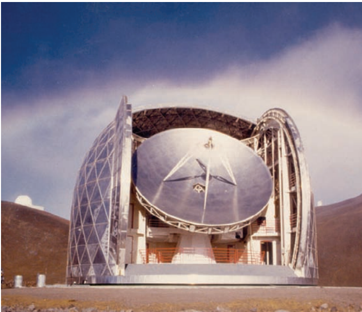
Fig.1.8. The 10 m diameter CSO submillimeter wavelength antenna on Hawaii. (Submillimeter Observatory, California Institute of Technology)
