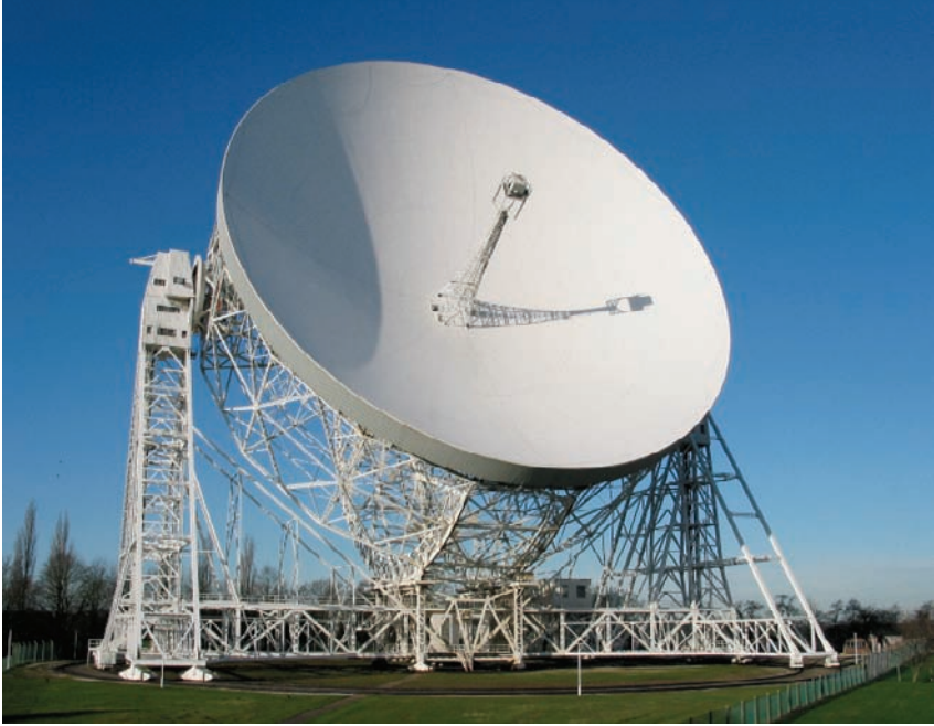
Fig.1.3. The 76 m diameter Lovell radio telescope at Jodrell Bank Observatory, England. The antenna has undergone two major upgrades, including a new, more accurate surface with a larger focal ratio. The central post to support the feed has been maintained. (I. Morison, Jodrell Bank Observatory)
